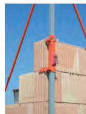
1. Sliding piece with chalk line support, level and angle adjustment system
