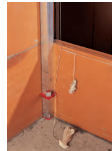
Spring-mounted pedal
